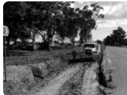
Road upgrading within the Delatite Shire.
