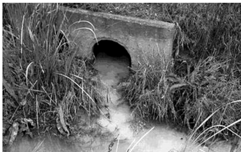
Greywater flowing into an open waterway.
