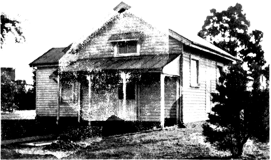
Edenhope Courthouse (1897). Closed on 1 January 1983. Building is currently unoccupied and in poor condition.
