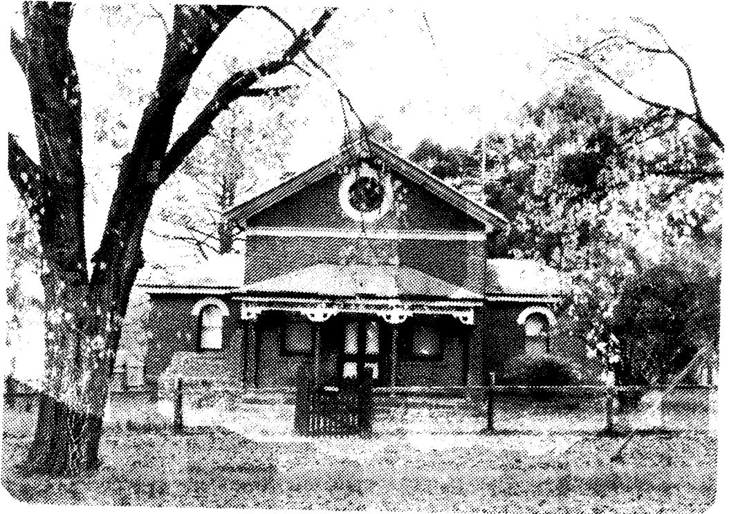
Fryerstown Courthouse (1879). Building is classified by National Trust and is now privately owned.
