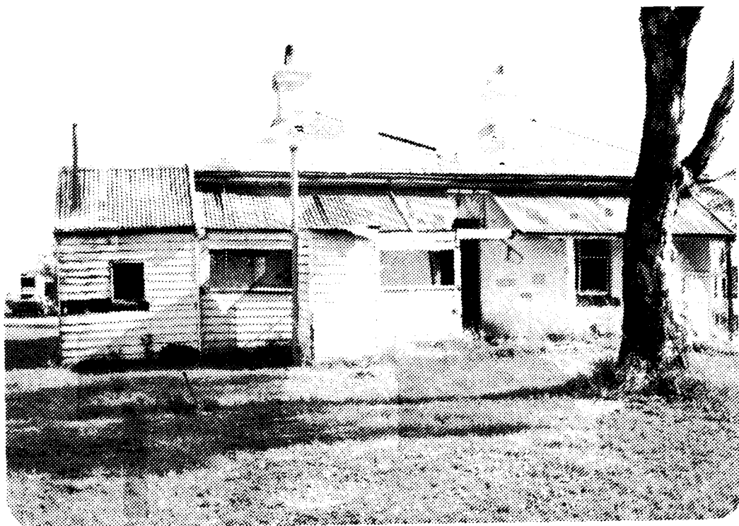
Rear of derelict former police residence adjoining Avenel Courthouse. The former Lands Department granted free use of the building in 1969 to the local Historical Society to establish as a museum.
