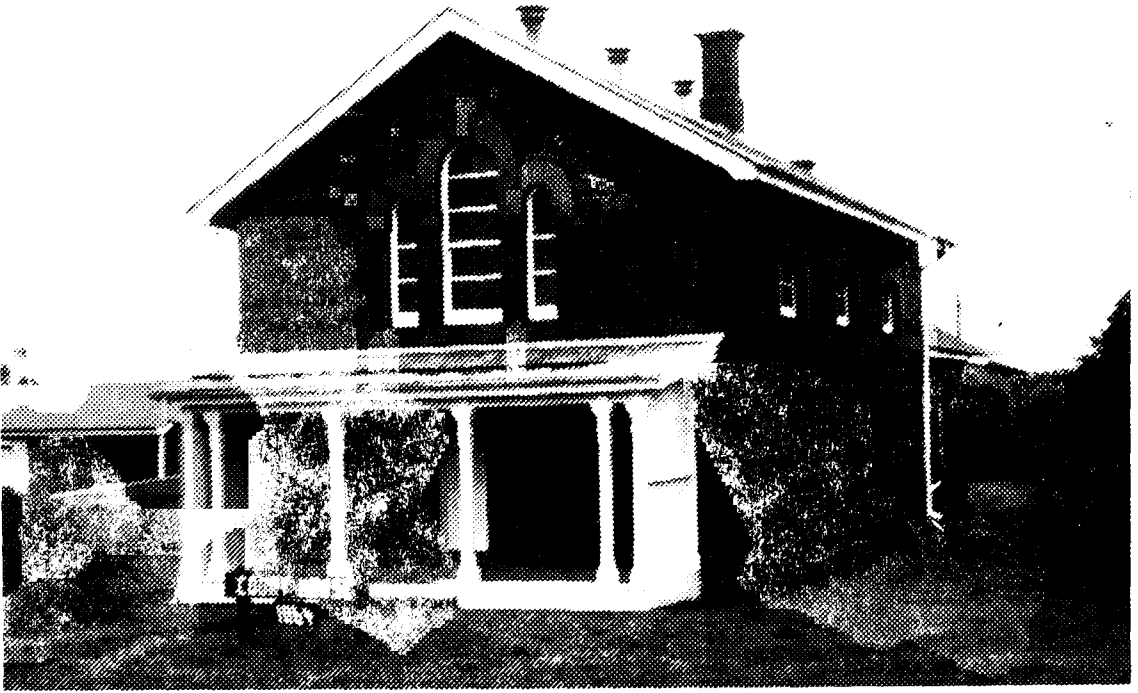
Mortlake Courthouse (1864). Closed on 1 January 1983 and currently managed by local Committee, in association with National Trust.
