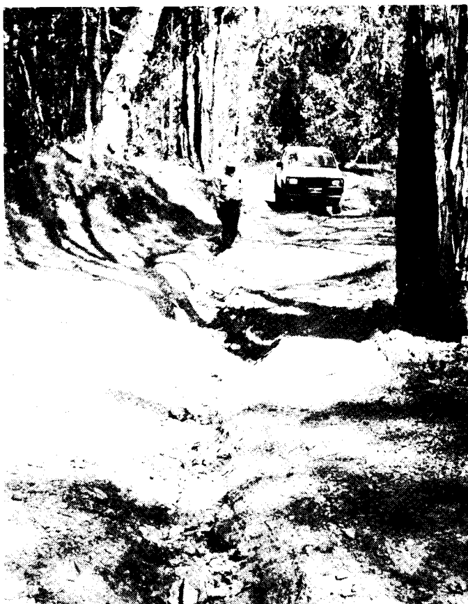
(Left) A deeply guttered and washed out track in the Alexandra region.
