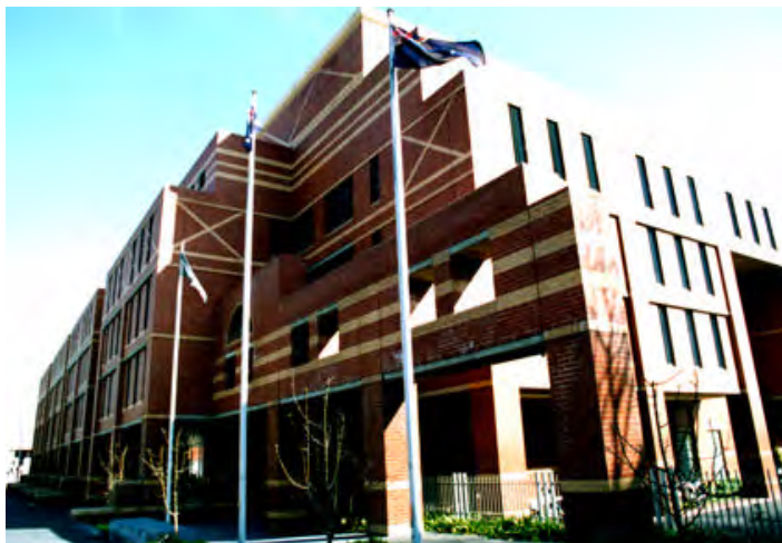
The Melbourne Assessment Prison, a CORE prison located in West Melbourne.
