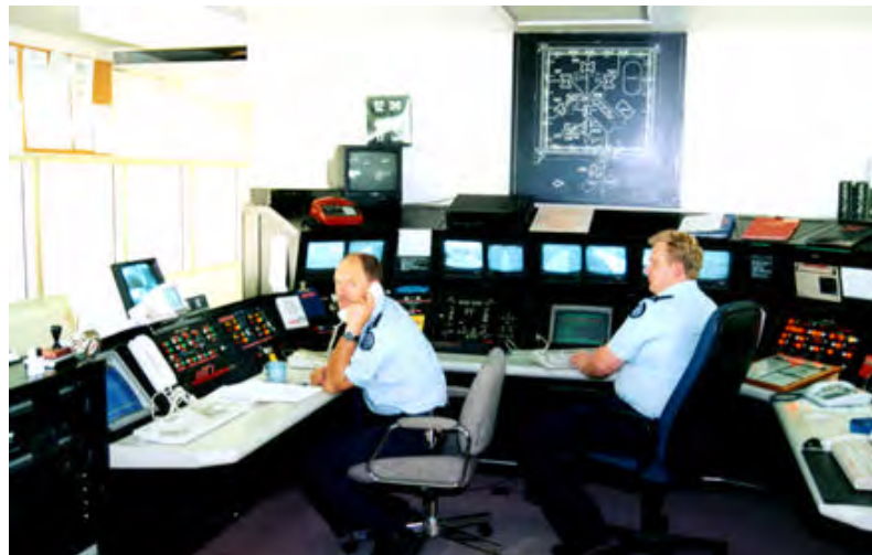
Electronic surveillance facilities in the control room of Barwon maximum security prison.
