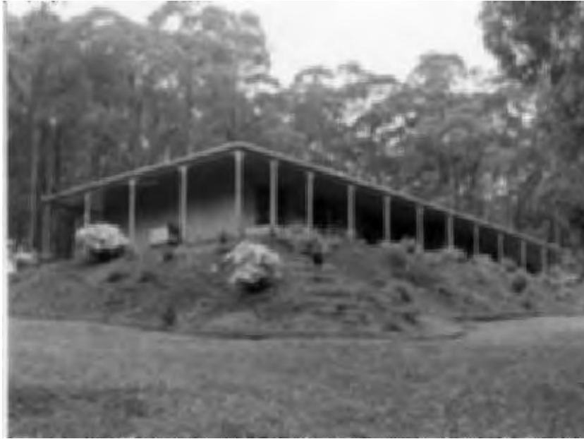
Effective planning controls can ensure that new homes in interface areas are designed and landscaped to minimise the wildfire risk.
