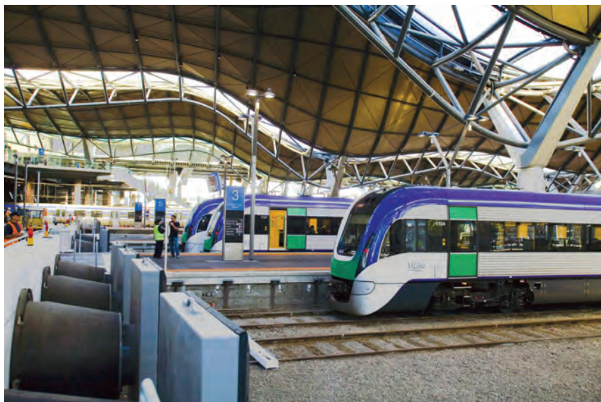
An internal view of the regional rail terminal.
