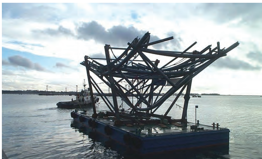
A section of the station's wave roof being transported by barge during the construction phase.
