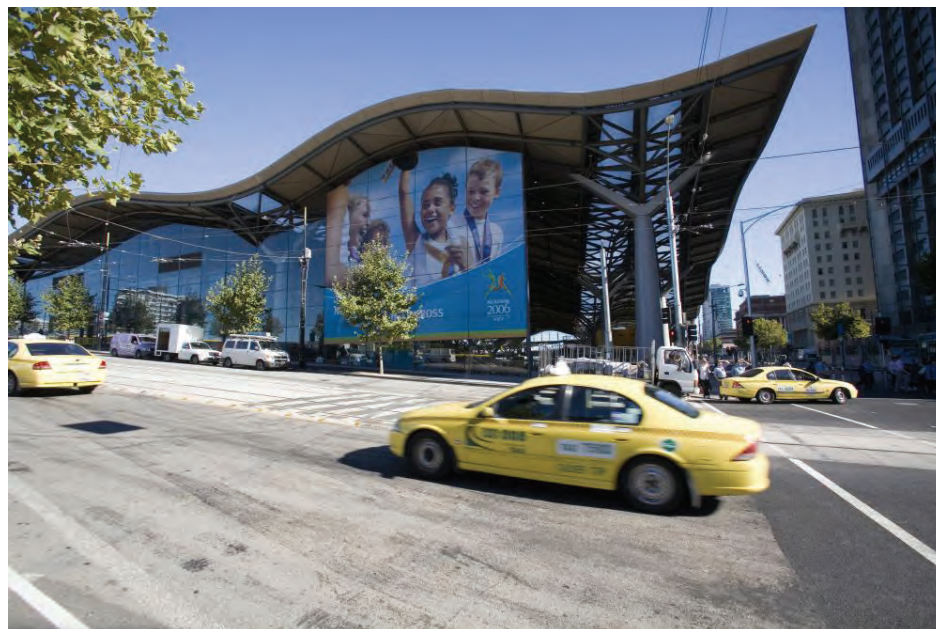
In March 2006, the station was ready for the Commonwealth Games.
