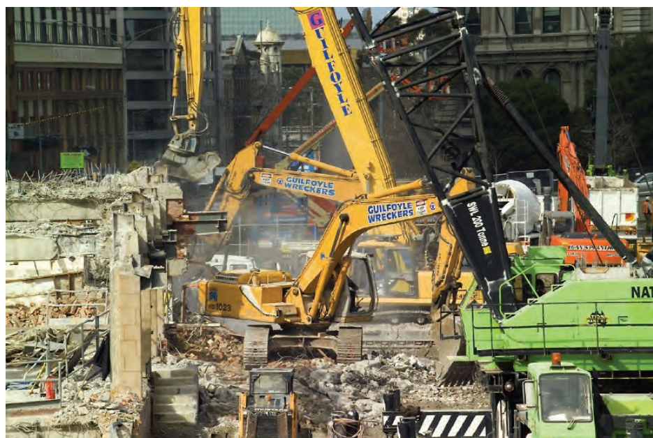
March 2004 saw the closure and demolition of the old station building.
