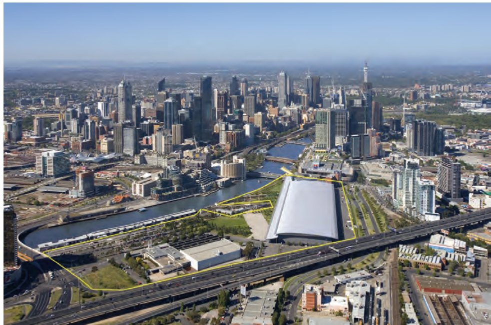
Aerial view of the Melbourne Convention Centre Development site.
