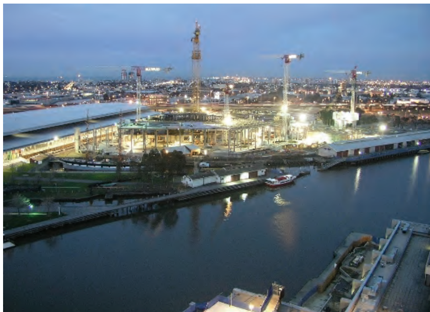
Image showing the progress that the MCCD was making in August 2007.
