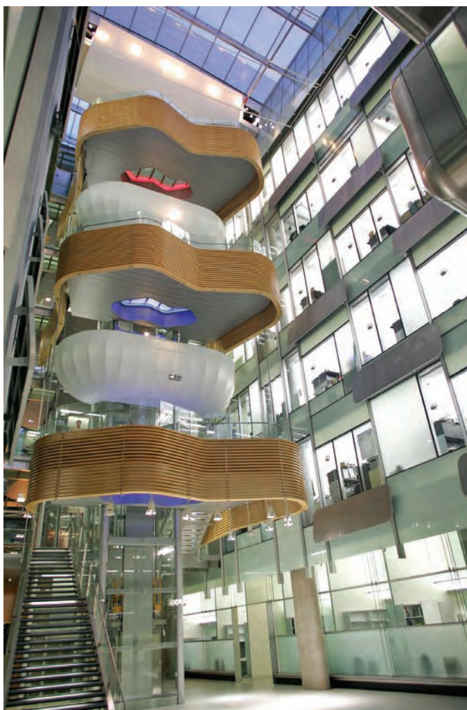
The internal atrium of the Bio21 Institute building. Photo provided courtesy of the Department of Business and Innovation.
