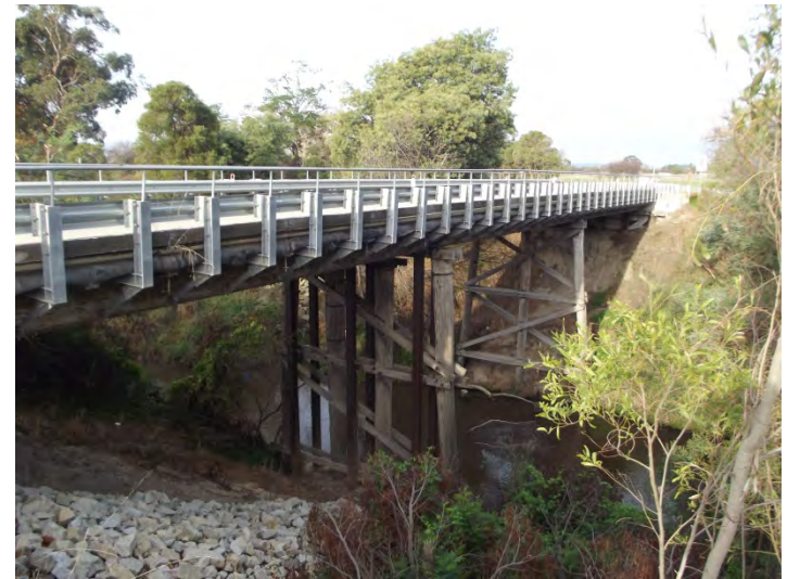
Bridge in Cardinia. Photo courtesy of Cardinia City Council.
