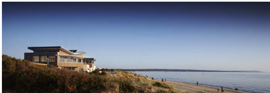
Carrum Foreshore and Lifesaving Club. Photo courtesy of Kingston City Council.
