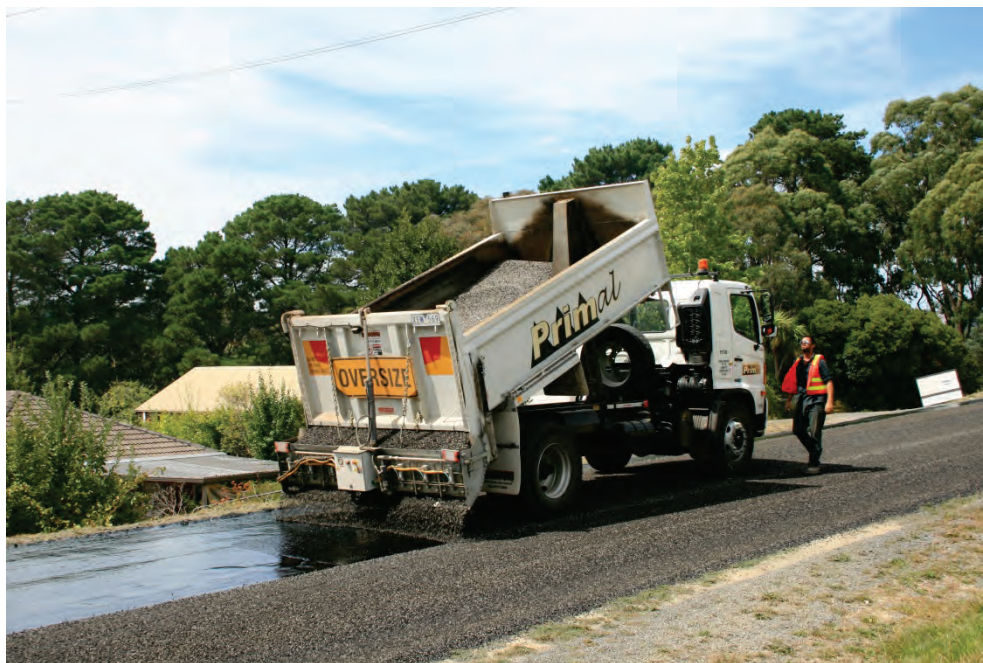
Road sealing, photograph courtesy of Hepburn Shire Council.
