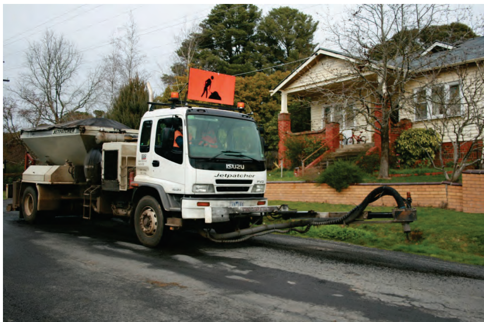
Road repairs, photograph courtesy of Hepburn Shire Council.
