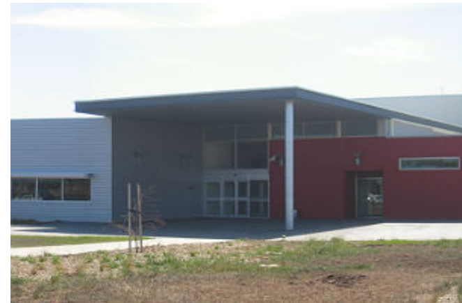
Tarrengower Prison (top) and Marngoneet Correctional Centre (bottom). Photos courtesy of Corrections Victoria.
