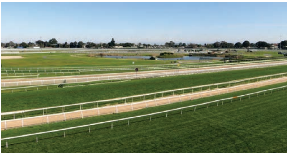
Encroachment of fencing on the reserve.
