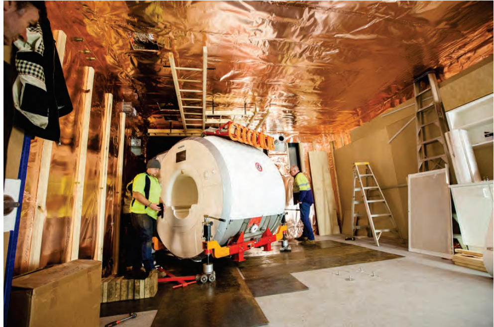
Installation of an MR scanner. Photograph supplied by Alfred Health Radiology.
