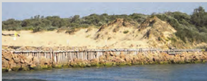
Left: Lakes Entrance training wall, showing the rock protection failing.
