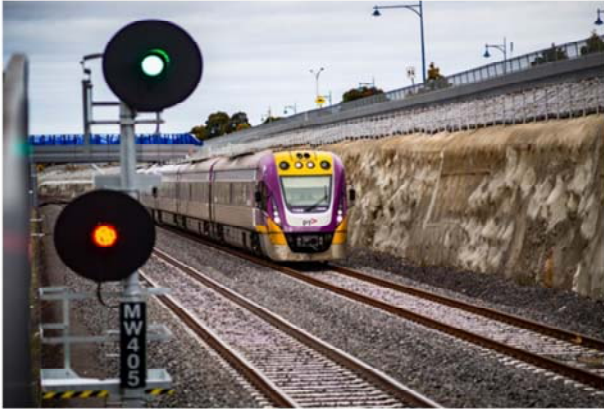
A rail cutting designed to reduce train noise on the approach into Wyndham Vale Station. Photograph courtesy of DEDJTR.
