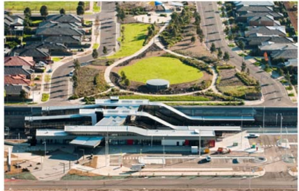
A new station was constructed at Wyndham Vale as part of the RRL project. Photograph courtesy of DEDJTR.
