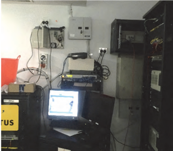
Public safety CCTV system Network Video Recorder equipment kept in an unlocked rack located in an open staff work area.
