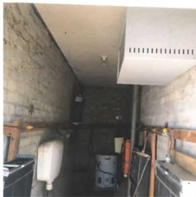
CCTV system cabinet hosted in the maintenance room for a public toilet in a dusty environment without any temperature or humidity controls.
