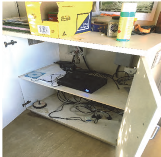
Digital Video Recorder kept inside an unlocked wooden cabinet without any environmental controls.
