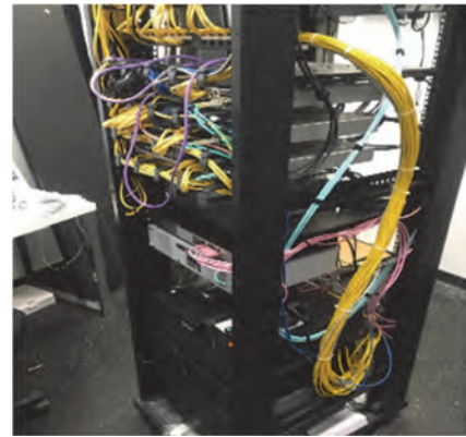
Network Video Recorder equipment kept in an unlocked rack with disorganised cabling.
