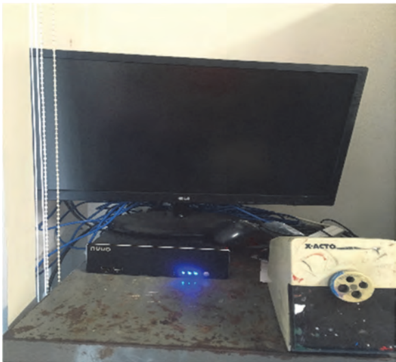
Digital Video Recorder for a CCTV system kept insecurely on the top of an office locker shelf.
