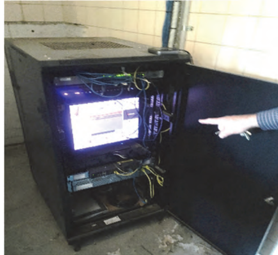
Public safety CCTV rack unlocked and hosted in the maintenance room for a public toilet, without any temperature, humidity or water detection controls.
