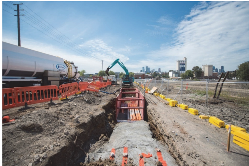
Utilities have been protected or relocated during the early works phase of the Melbourne Metro Tunnel Project. Photograph courtesy of RPV.
