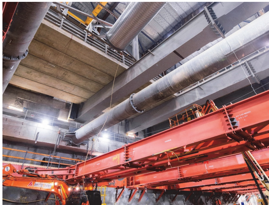
The access shafts at the State Library precinct originally used concrete and tubular struts (seen at the top of the photo) but this was later replaced with the orange modular steel struts requested by the PPP consortium. Photograph courtesy of RPV.
