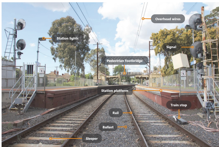
Figure 1E: Infrastructure assets on railways
