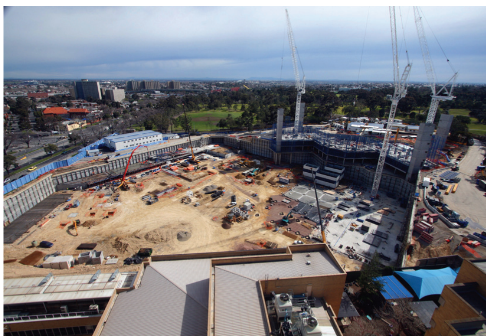
Excavation and early construction works at the new RCH site in August 2008.
