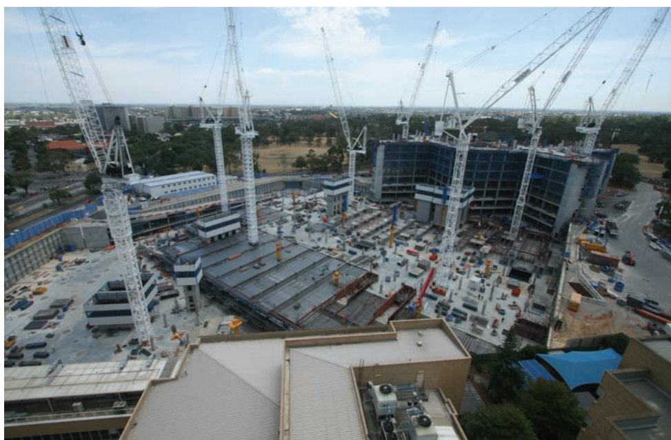
Construction progress on the new hospital in late January, 2009.
