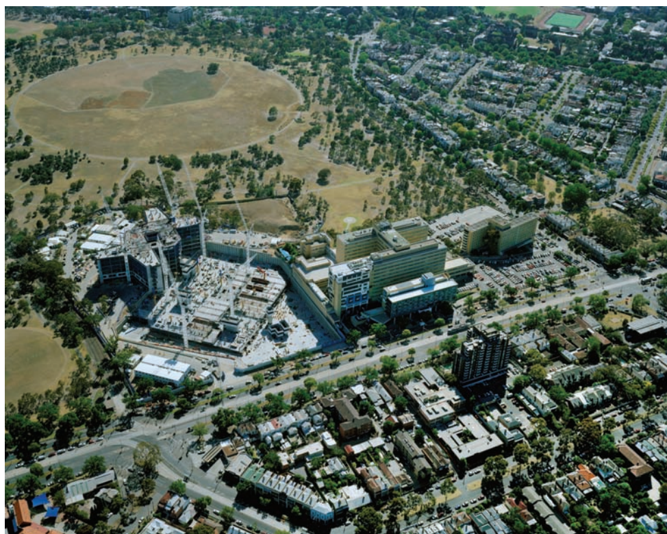
An aerial view of the RCH site, showing the new hospital under construction (left), and the existing hospital campus (right), which will be largely demolished and converted to parkland.
